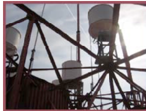
Job Site: TTI Tower Elevation: 990' Microwave Antenna Installation Completed
