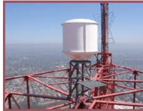
Job Site: TTI Tower Elevation: 990' Microwave Antenna Installation
